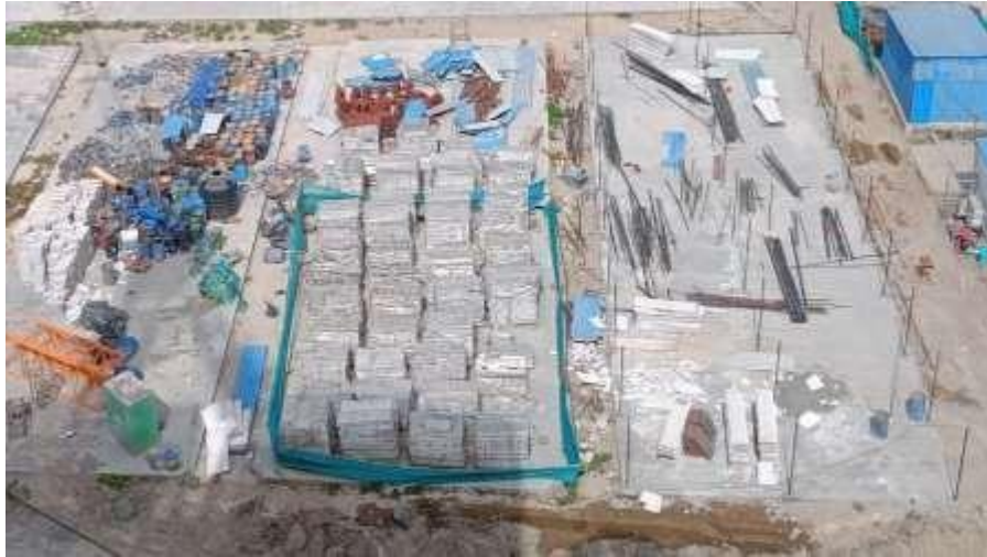
Figure 7: Set in order at site, Source: Joyville Manjari Yard (SPRE)
