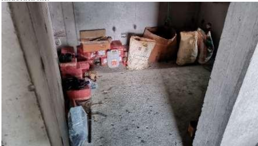
Figure 6: Effective use of Workfront logistic plane; Source: Joyville Manjari T9 (SPRE)
